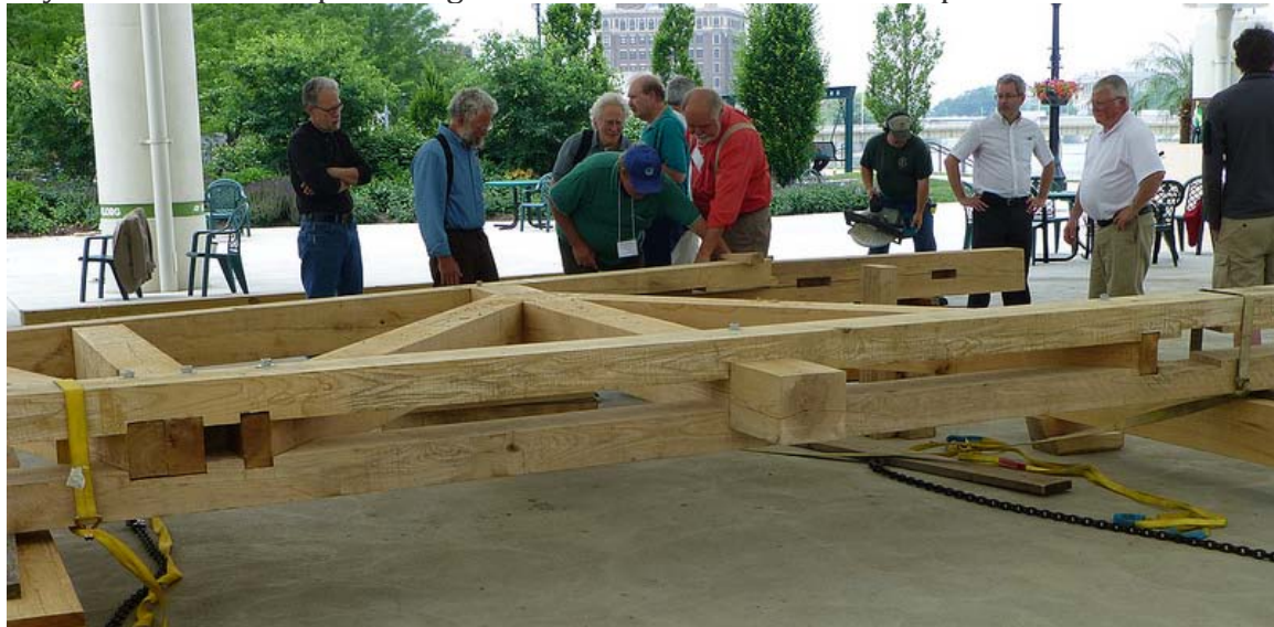
Dave Kirwin and Will Truax led a timber framing demonstration of a kingpost truss at RiverScape Pavilion on Dayton's Miami River waterfront.
