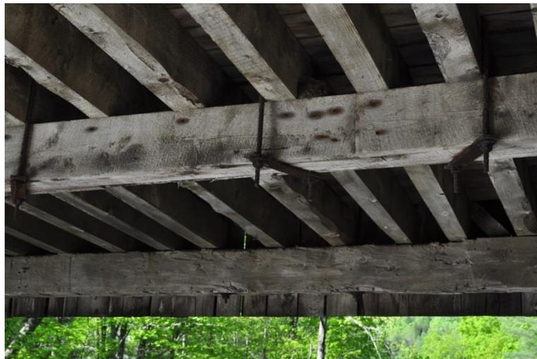
Fig. 12 Photo showing the condition bottom chord member of the Moxely-south truss
