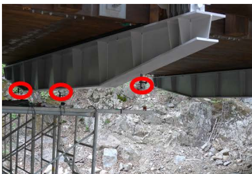
(a) Center cross beam
