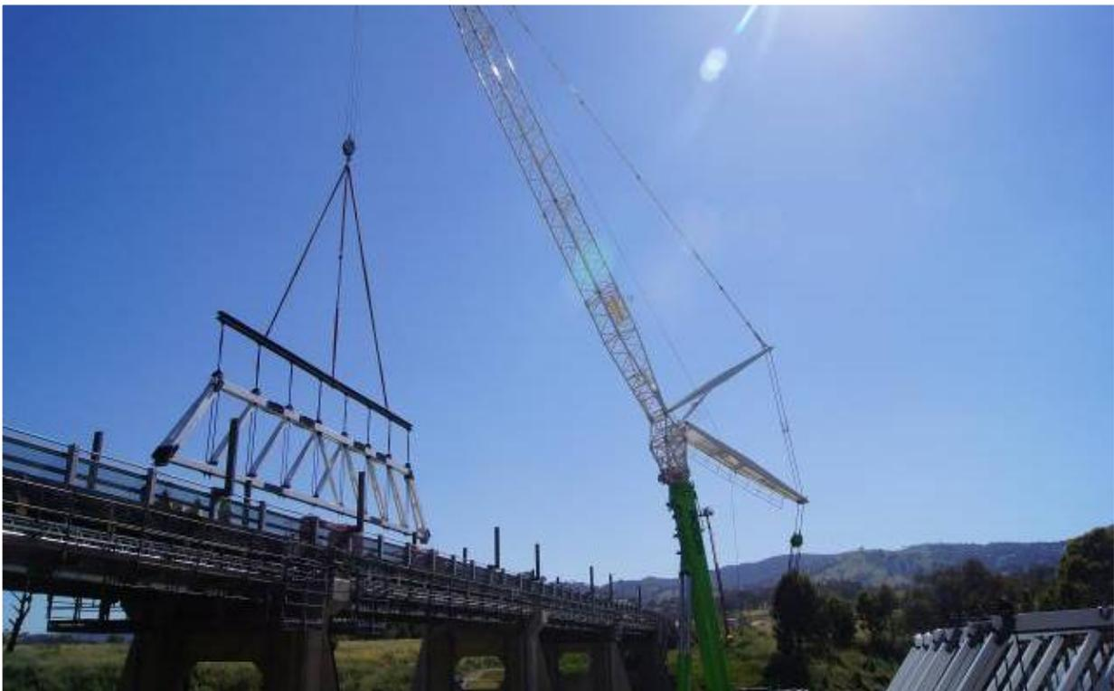
*Figure 10 – Truss being lifted into place using a 400t mobile crane*
