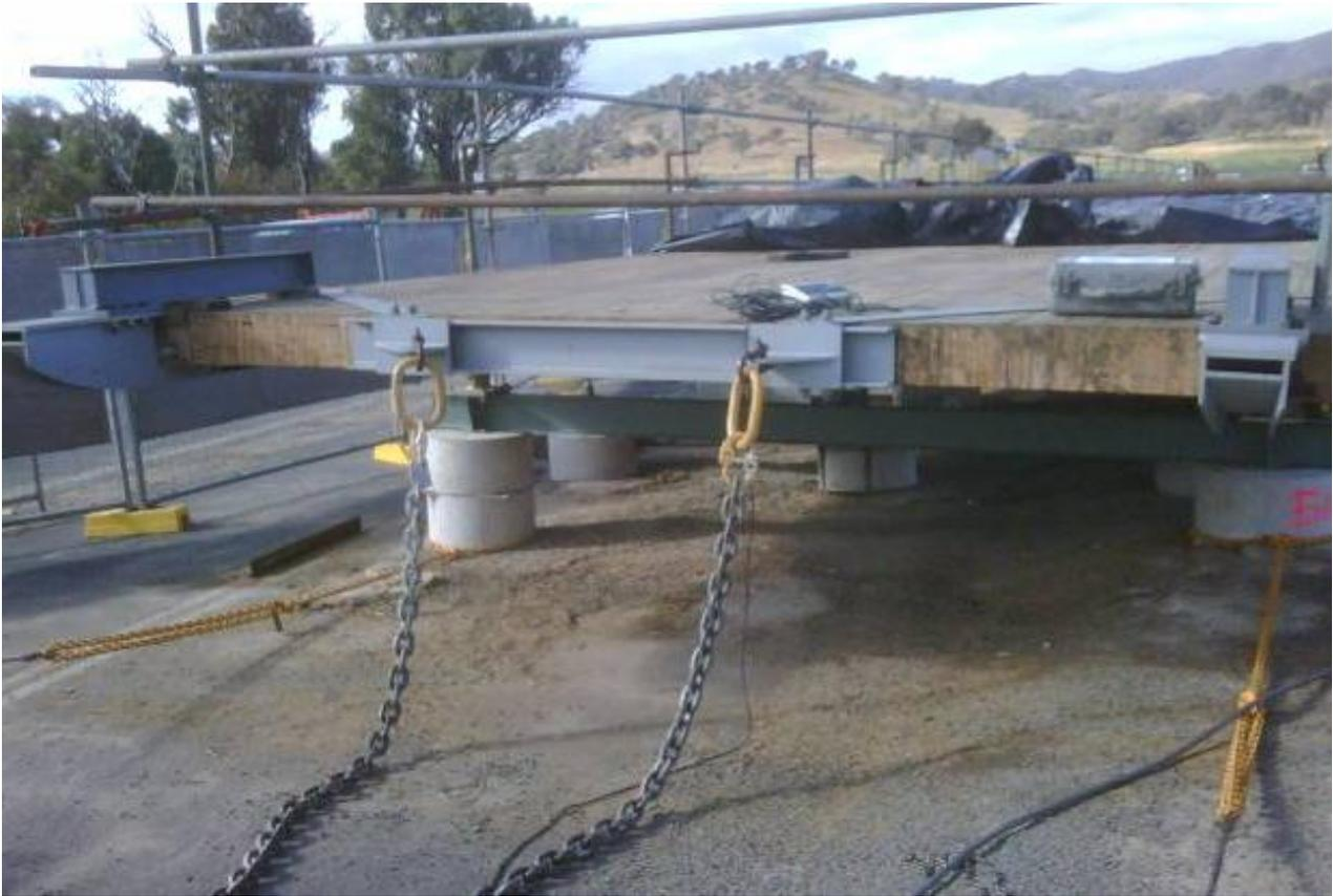
*Figure 13 – SLT deck Launching Nose*
