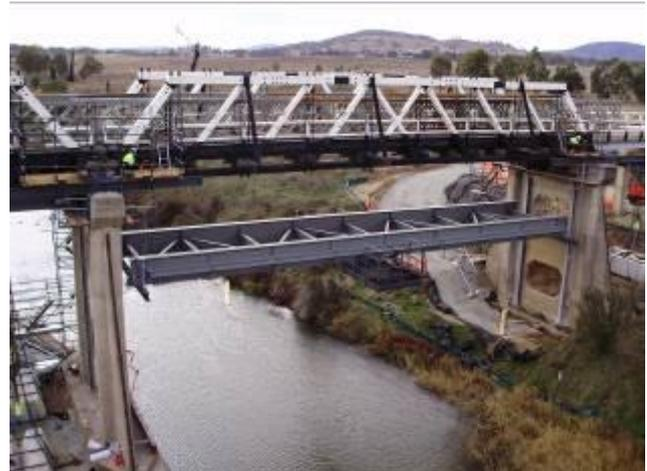
Figure 3 – Temporary support structure 2008
