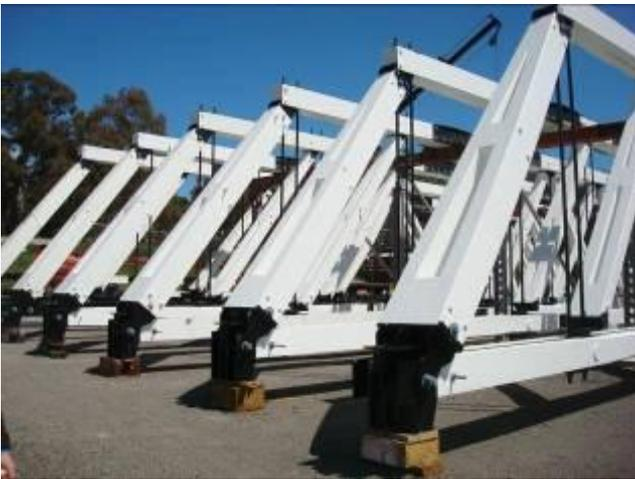
*Figure 8 – Truss Assembly on site*
