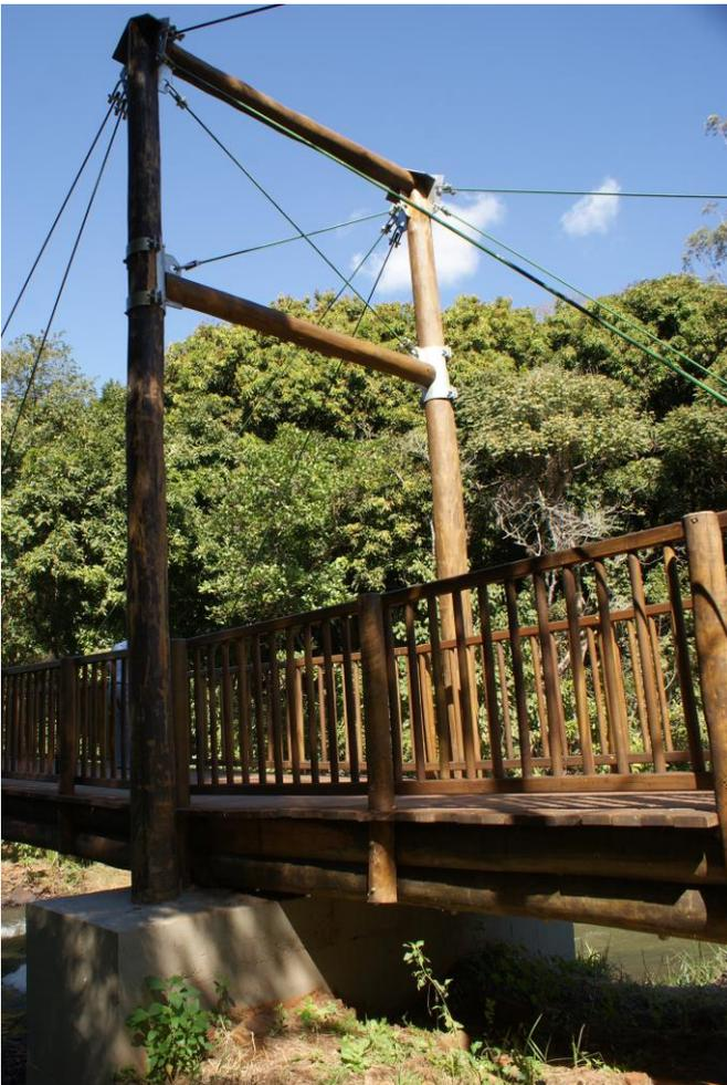
*Fig. 7 Foundation block and a tower poles composing of the footbridge.*
