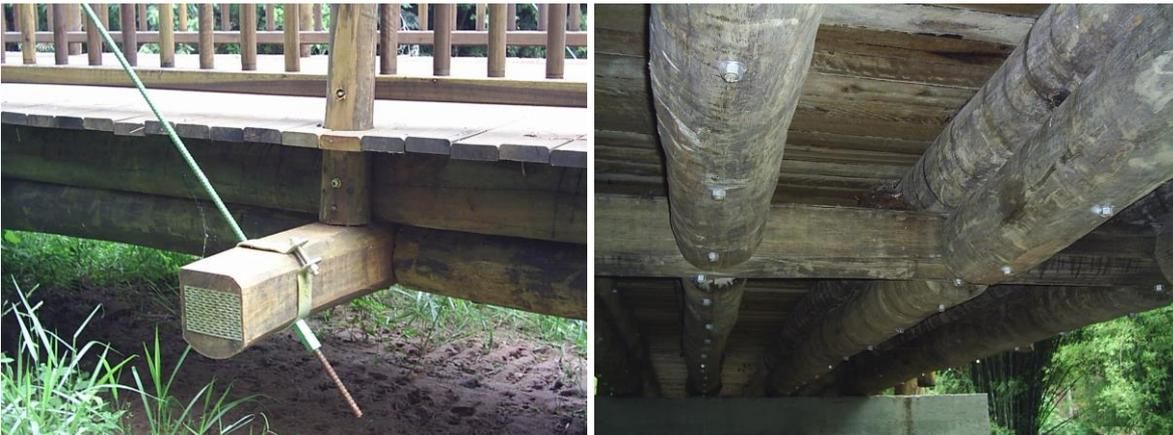
*Fig. 9 Connections are stayed the transversinas stringers and double pieces.*
