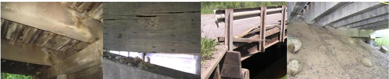
*Figure 4 – Visual inspection conditions including discoloration and staining, insect activity, mechanical damage and build-up of sand and gravel.*
