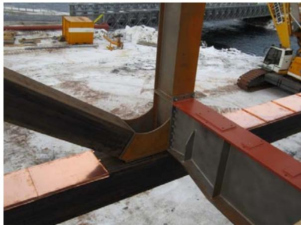
*Figure 8 Crossbeam/vertical connection*
