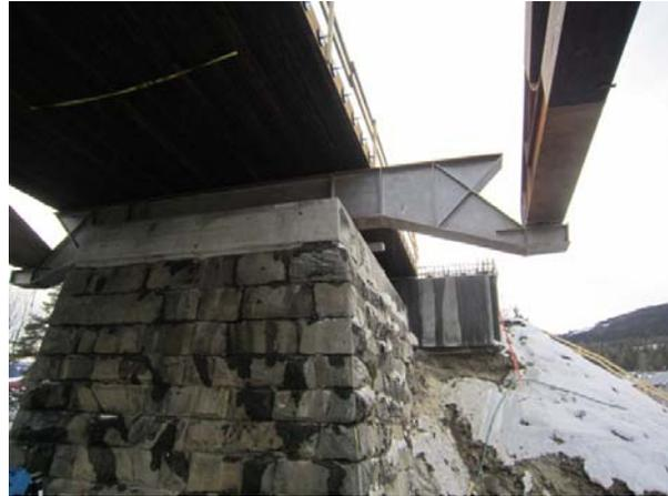
Figure 5 Truss support in axis 1
