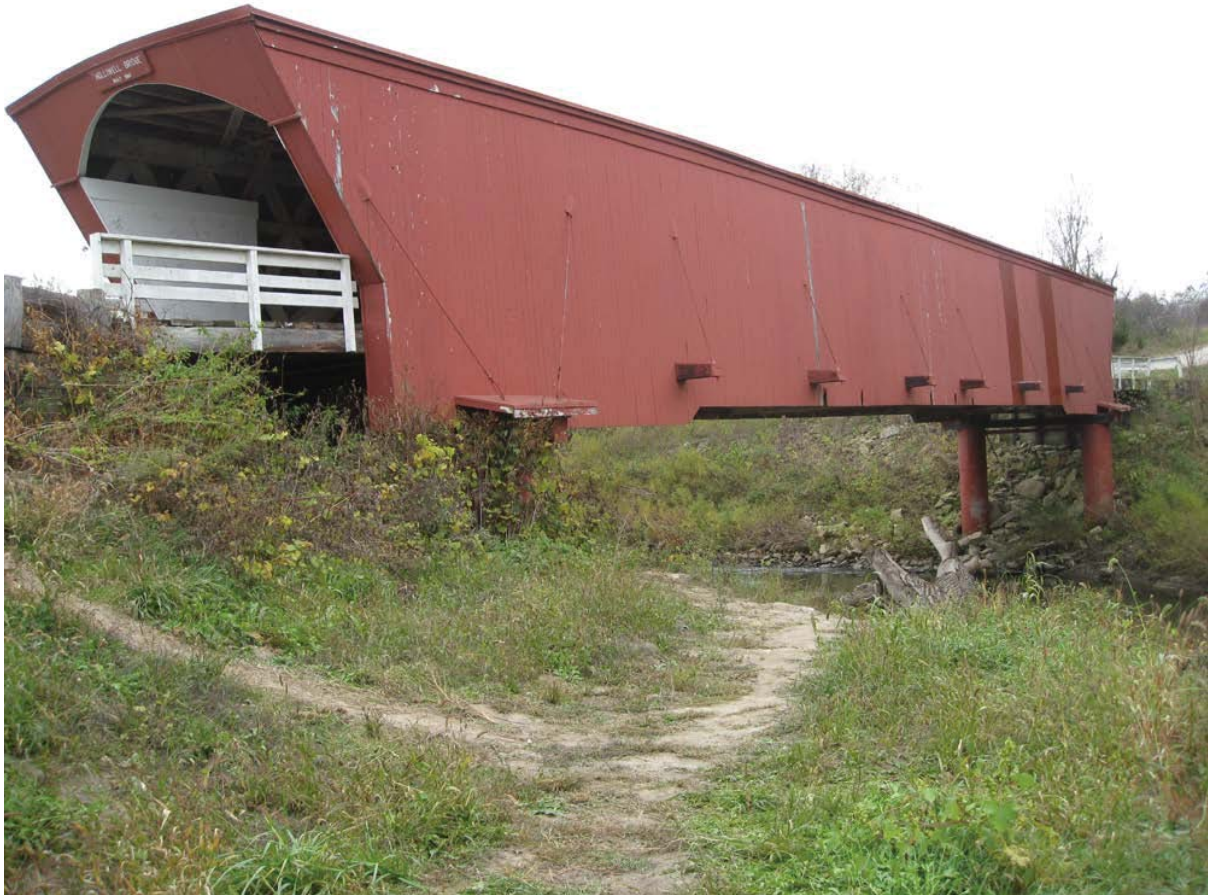
Figure 1. Holliwell Bowed Arch Covered Bridge in Madison County, Iowa.
